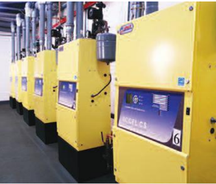
MULTI BOILER ARRAY
