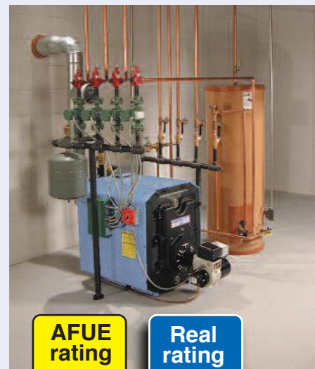
Typical high-mass boiler with indirect water heater.
