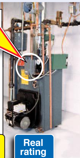
Cast iron tankless coil boiler.
