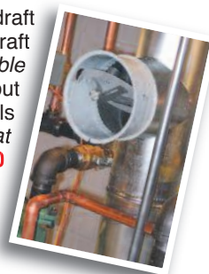
Conventional gas boiler and water heater.
