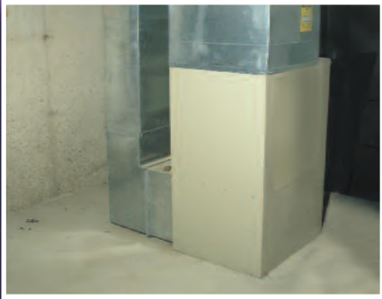
Hydro-air and heat pump backup
